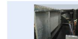
DX-coil (Direct expansion coil)
